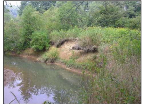
Eroding streambank along Redbank Creek
