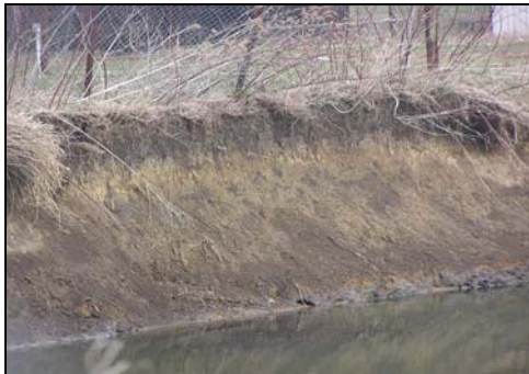
Severe erosion along a section of Buffalo Creek, resulting in significant loss of streambank each year
